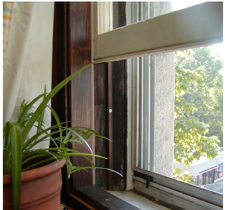
This window upgrade included truing sashes to fit the opening, adding leaf seals (see the white seal on the left, against the outside edge of the interior jamb trim), and routing in a beefy sill gasket.
