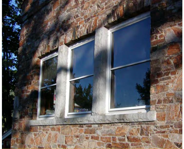
Although these original wood windows are fitted with conventional storm windows, the owner also wanted to upgrade the existing windows to work more smoothly and to be less drafty.
